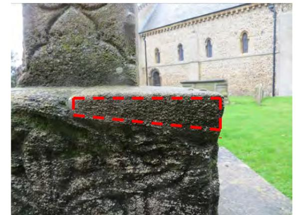
Photograph 24: Repair to shaft base
