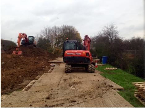
The works at Wagtail Drive involve landscaping a parcel of land adjacent to Drapers Farm Sports field to create two attenuation ponds. The ponds will be separated by a public footpath and a low flow channel. In addition, a hydro-brake will be installed to restrict the rate of which water flows into the downstream system.
